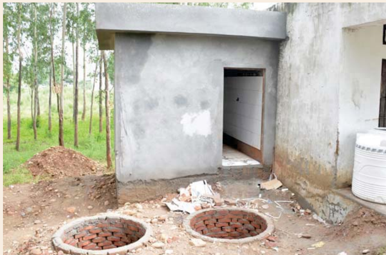
Construction of girls toilets in schools under Swacch Bharat Mission
