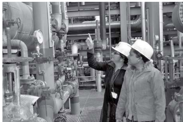
Engineers working at the Plant
